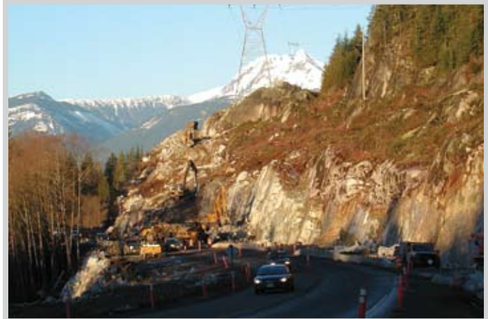
Crews begin removal of rock at one of the largest rock cuts on the project at Darrell Bay. The target is to remove 5000 cubic metres (equivalent to 33 railway boxcars) of rock each week.
