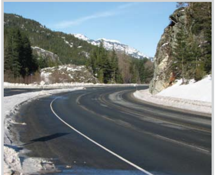
The new Cheakamus to Rubble Creek section has improved pullouts, 5 km of new passing lanes, wider shoulders and improved sightlines.
