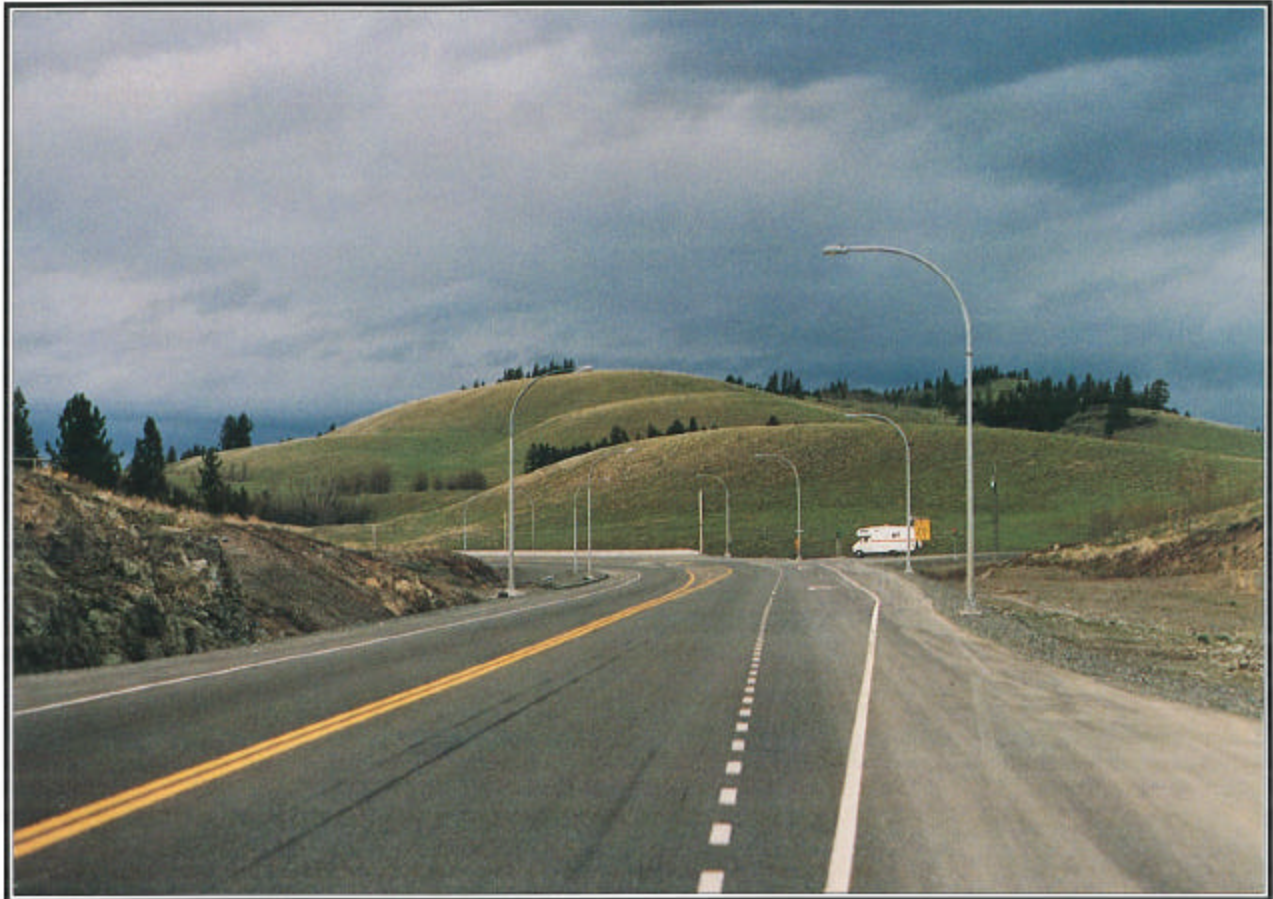
Above Ground Utilities
