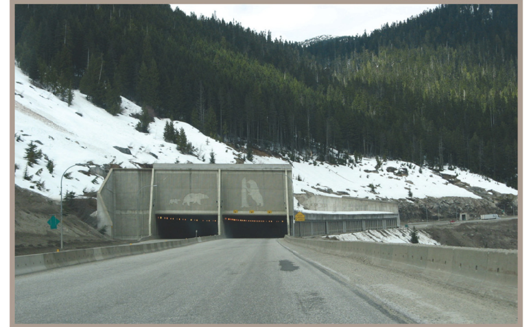
Hazard protection sheds will protect against snow avalanche and rock fall hazards.
