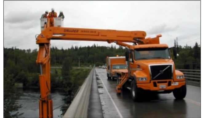
The Ministry of Transportation Snooper truck in the process of inspecting the Stuart Bridge near Fort St. James. In the bucket are Chris Thornhill, Mike Rutledge, and Jen McConnachie.
