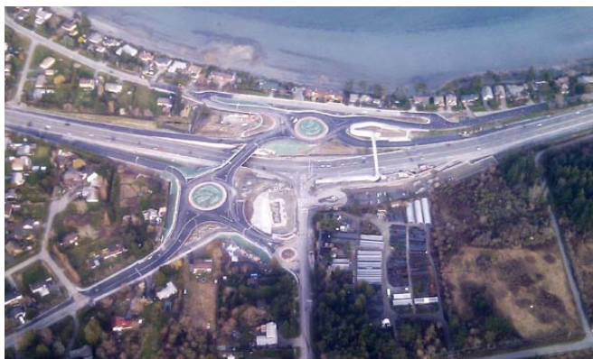
Aerial view of the new Highway 17/McTavish Interchange
